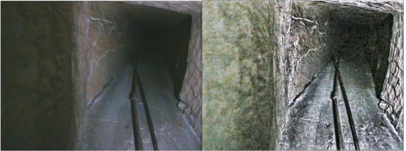
Diagram I-18 - the obviously rotated middle section of shaft
